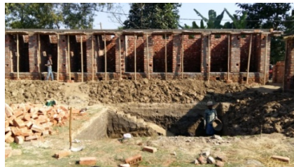
(DGSC Under Construction)
