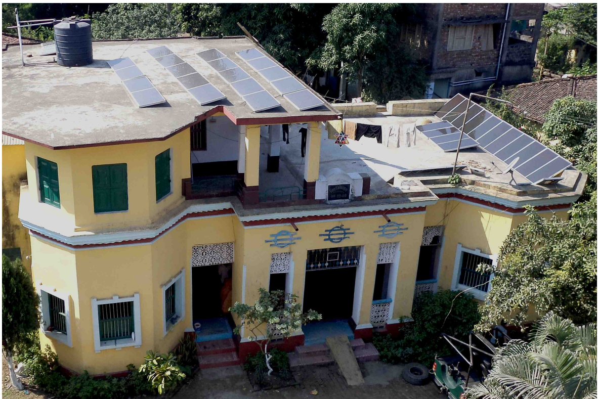
(A solar PV rooftop system runs DESI Power's head office in Araria)
